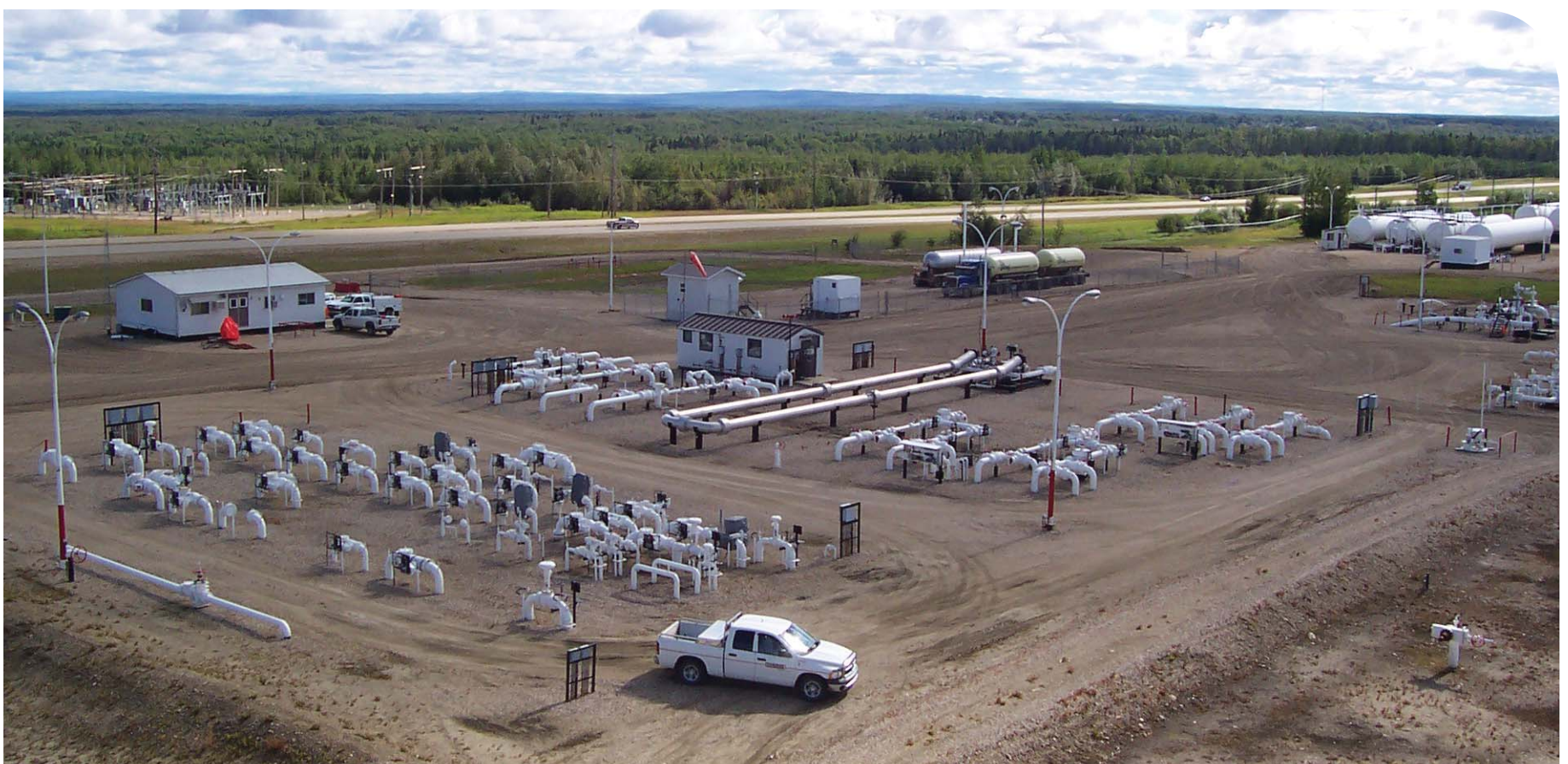
Pembina's Fox Creek Station will receive a few modifications and increased storage capabilities as part of the Saturn Project.
